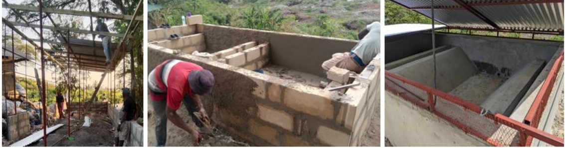
Figure 6: Construction of the compost cage and waste sorting collection station
