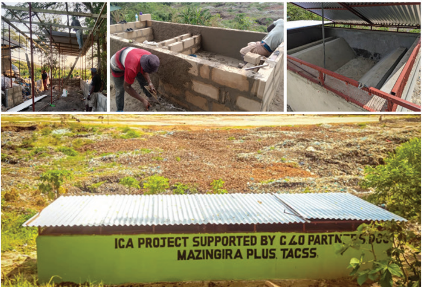
Figure 6: Construction of the compost cage and waste sorting collection station
